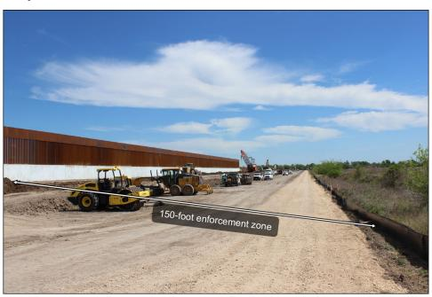
Figure 2: Border Barrier and Enforcement Zone under Construction in Rio Grande Valley Sector
